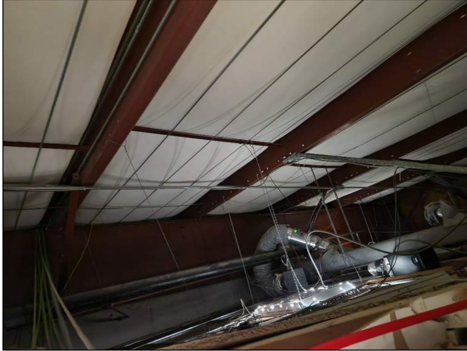
Pre-Engineered Metal Roof Purlins and Bent.
