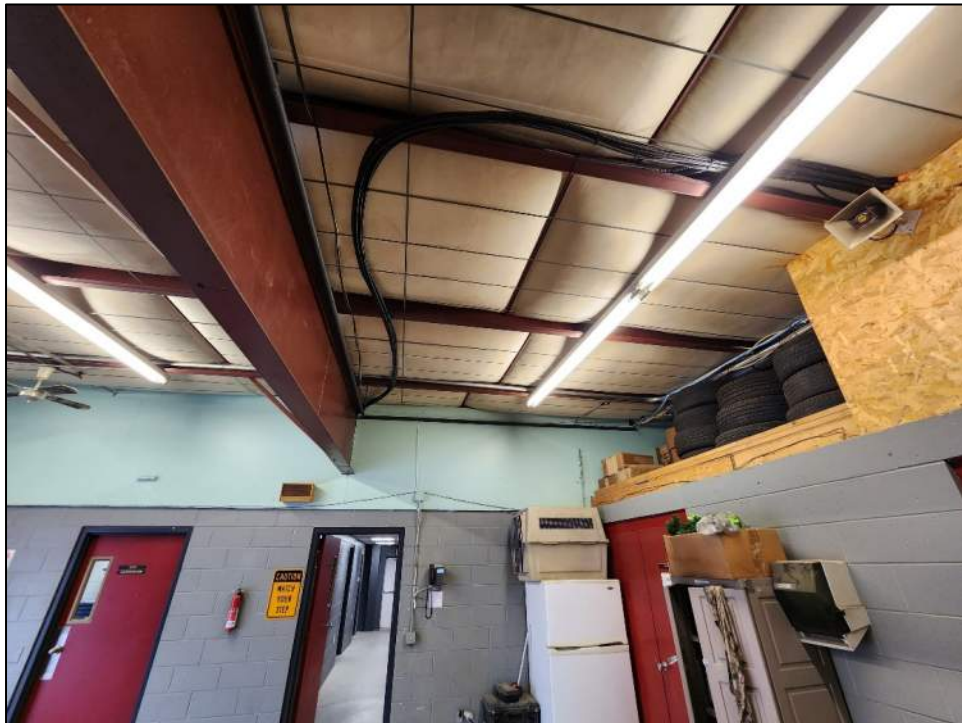
Pre-Engineered Metal Roof Purlins and Bent.
