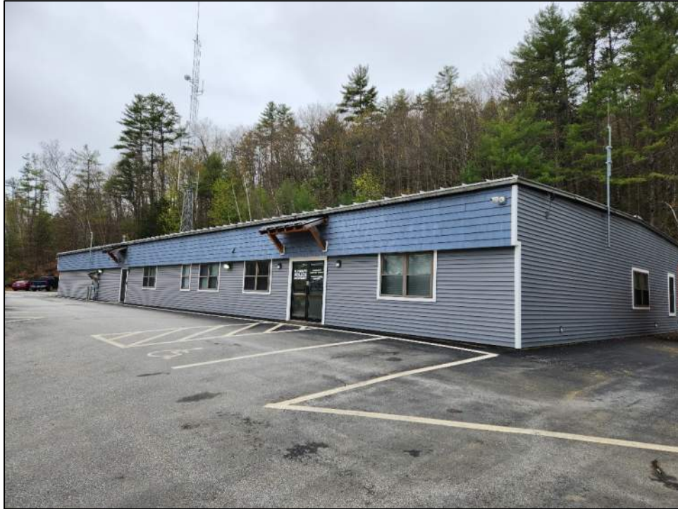
Front (East) Elevation.
