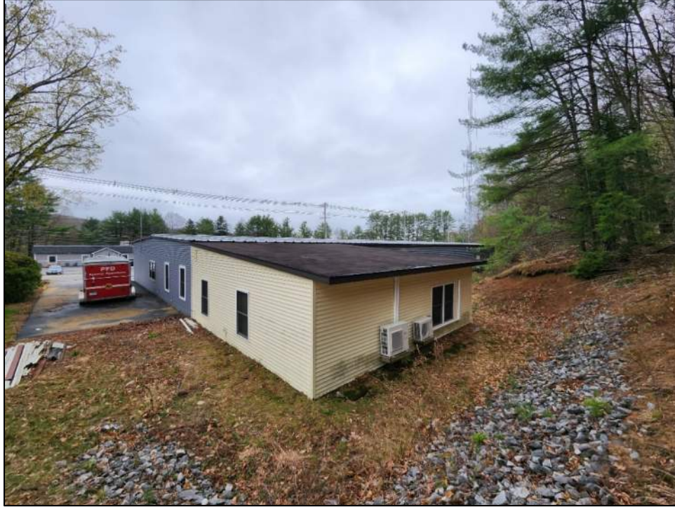
Side (North) and Rear (West) Elevations.
