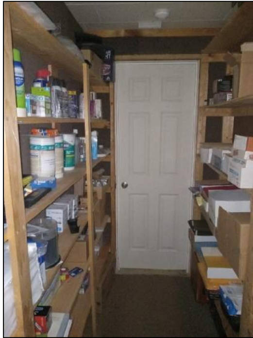
Unfinished Interior Closet Walls – Wall Framing Exposed.
