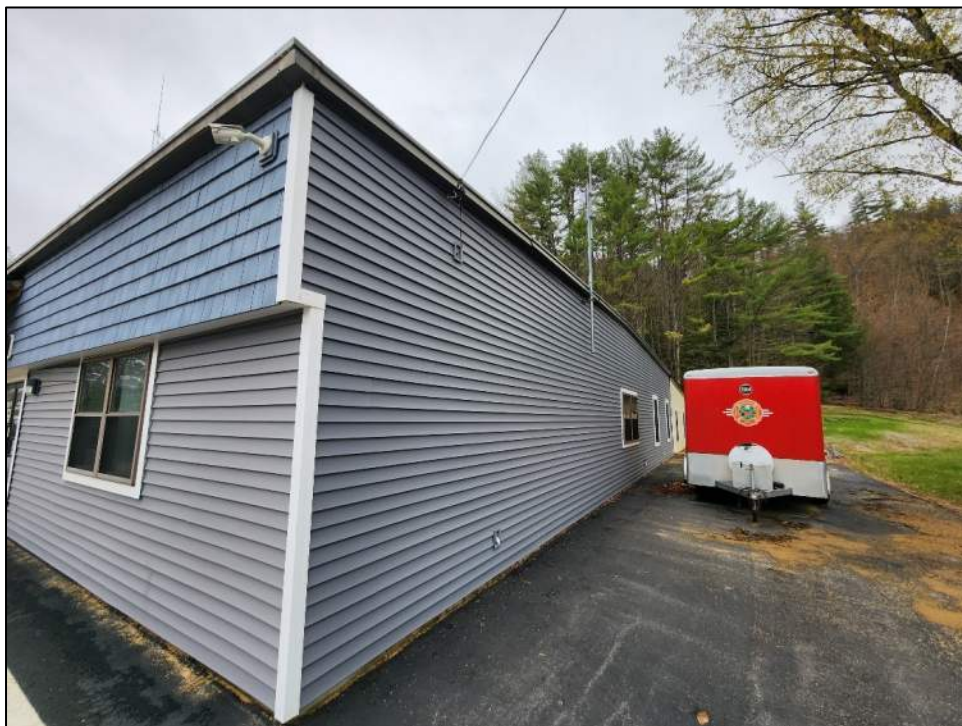
Side (North) Elevation.
